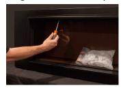
Locate screws holding in the glass and remove
